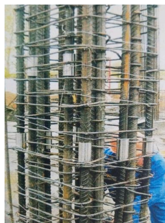
Fig. 6. Mechanical connections of LENTON reinforcement bars of the column
