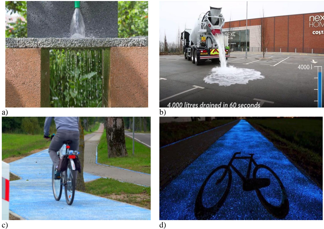
Figure 3. Upcoming types of coating for bicycle paths: a – permeable concrete covering; b – permeable asphalt covering; c – coating with a phosphor in the afternoon; d – coating with phosphor at night
