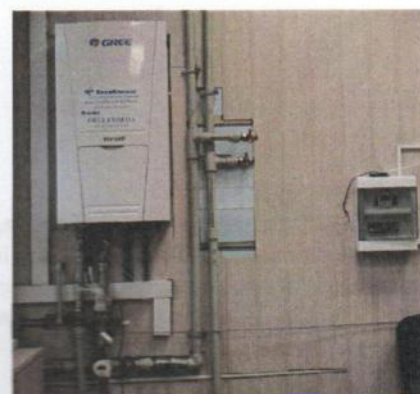
Fig. 17. Exterior view of heat pump of the split type "air – water" with heat output 6 kW
