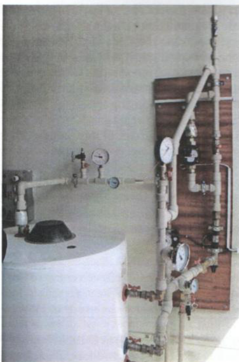
Fig. 18. Bivalent water heater-accumulator with capacity 300 l
