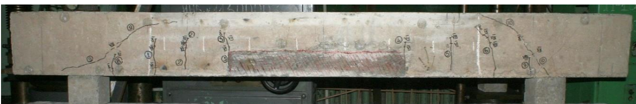
Fig. 4. Cracks in the sample RCD5
