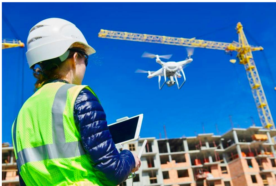
Fig. 2. Drones are Revolutionizing High-Rise Construction
