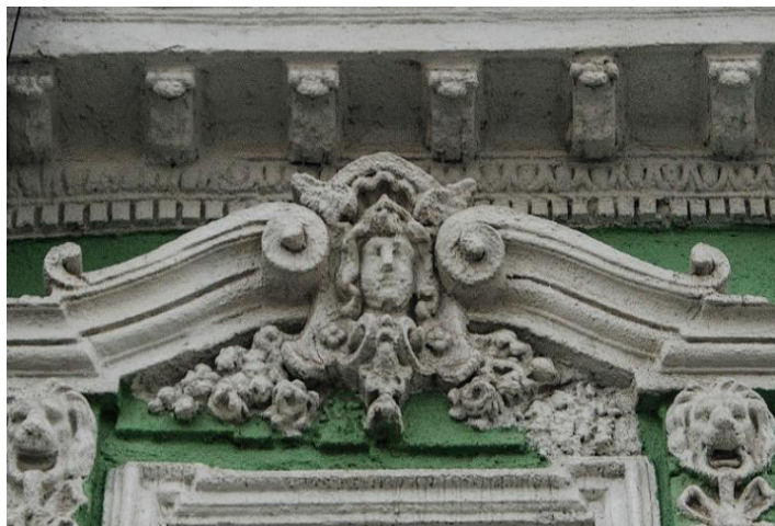
Fig. 10. Mercury on the facade of the house
