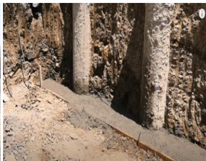
e – concrete foundation is performed
