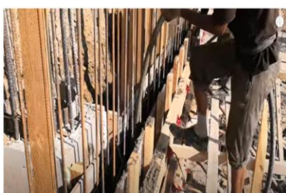
h – concreting process
